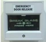
White MCPs are usually associated with the security system and are designed to unlock electronic door locks. Once activated the lock should disengage so the door can be opened manually. In most instances the activation of a security MCP will also activate the security alarm and send an alarm signal to the security monitoring company.
